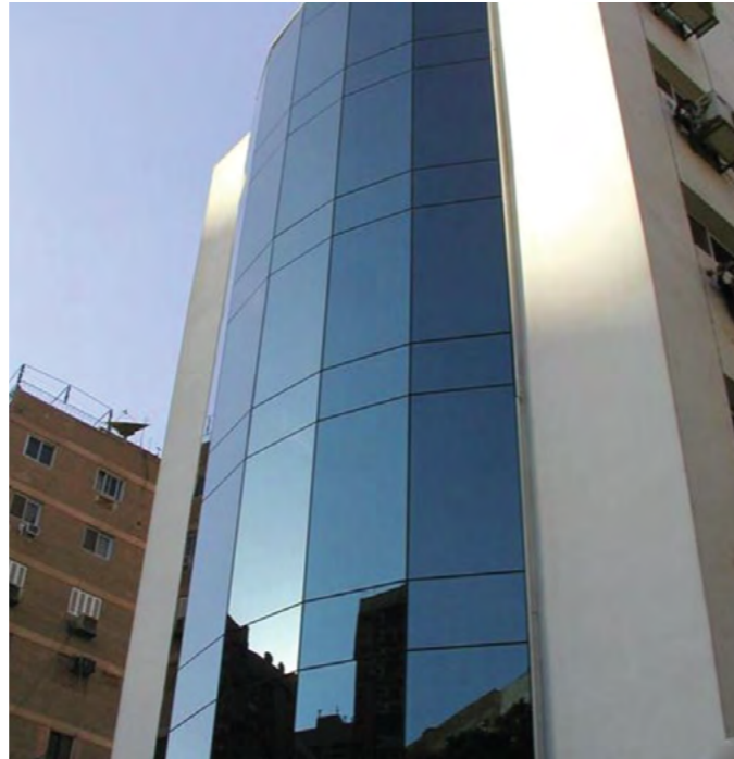
Security film UNICEF Facility, Cairo Egypt
